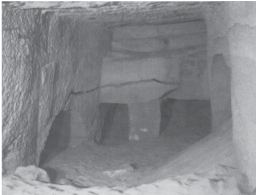
Figure 2: A general view of the false end. There is a modern buttress built under the bench in the middle of the Main Passage to support the bench.
